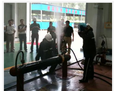
WITNESSED PRESSURE TEST
